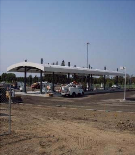
September 8, 2007 - Construction continues on the new Arco gas station.
