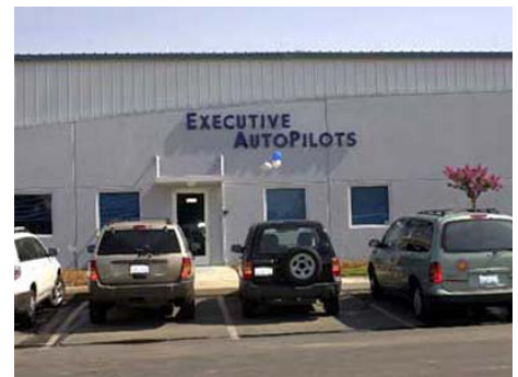
Executive AutoPilots hangar at Executive Airport.
