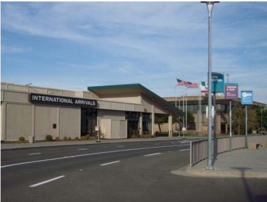
September 2006 - The International Arrivals building at Sacramento International Airport, where the airport's customs facilities are located.
