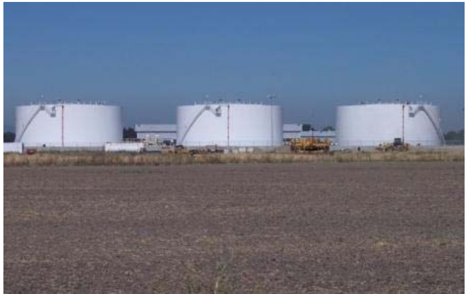
December 2005 - Three new fuel tanks at Sacramento International Airport. Photo by Paul Bennett.
